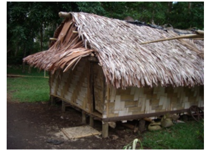
Our accommodation was a traditional village dwelling. Split bamboo woven together for the walls, strips of palm laid on short posts for the floor, and a thatched roof
