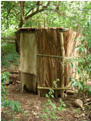
A “bush-toilet” - basically a Port-a-Potty sized structure with a one square-foot hole cut out of the floor, placed over a deep trench
